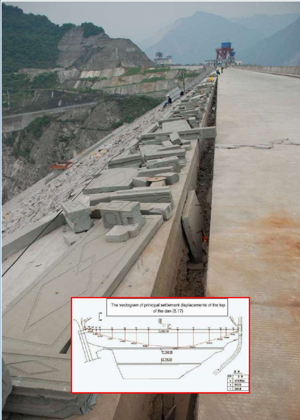
Fig. 1 Sliding failure of an earth dam
