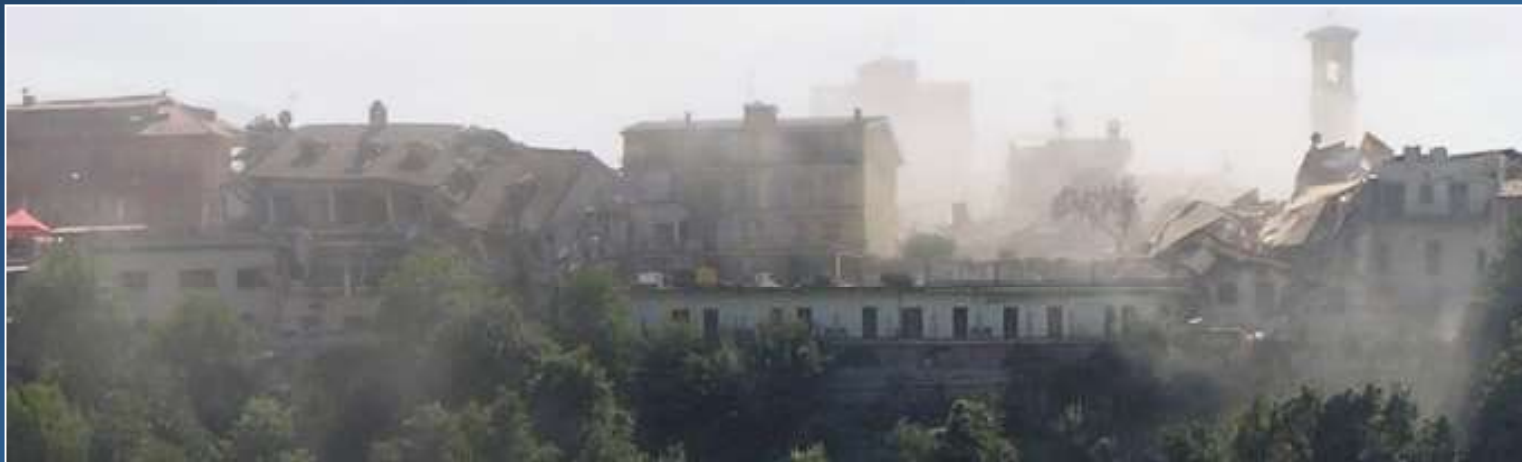
Photo taken on 2016.08.25 during an Mw 4.3 aftershock
