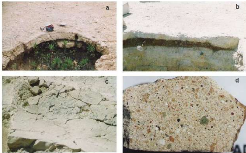
Figure 1. Photographs of general views of plasters: a) Floor from Kissonerga-Mosphilia; b) floor from Kalavassos-Ayios Dhimitrios; c) water channel from Kalavassos-Ayios Dhimitrios; and d) sample from the channel of Figure 1c (color figure available online).
