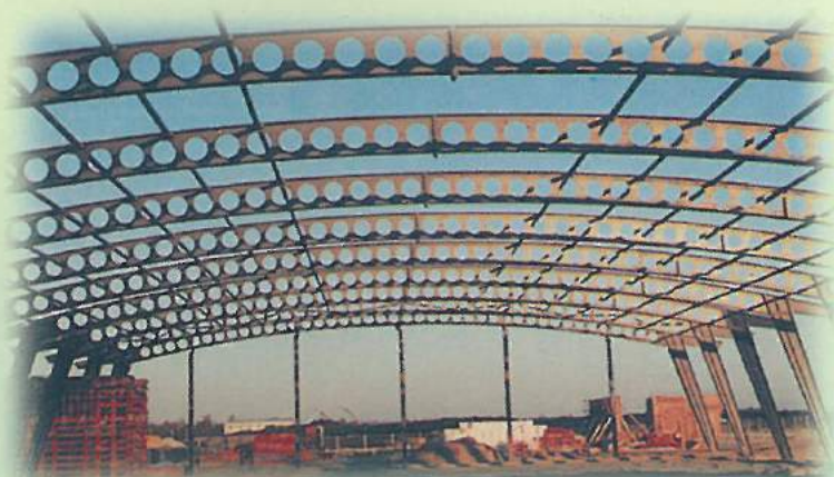
Curved roof span : 28m, Radius: 62m
