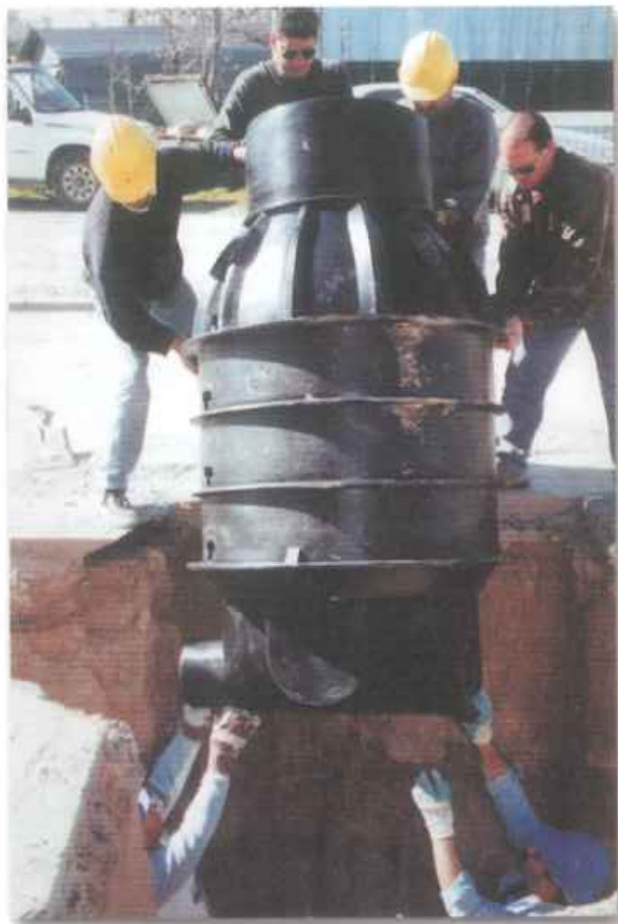
Installing ROMOLD "Combi" one-piece chamber in Limassol sewerage project.
