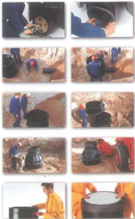
Installing ROMOLD "Combi" one-piece chamber in Limassol sewerage project.
