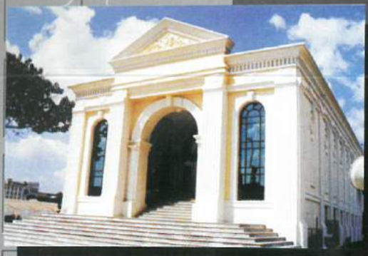
GRC Used in decoration of the building
