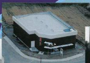
Germanos Main Offices & Distribution Center
