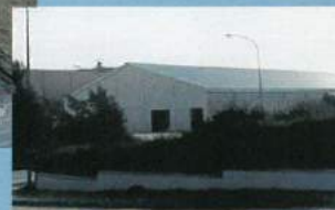
Zorpas Bakeries Factory
